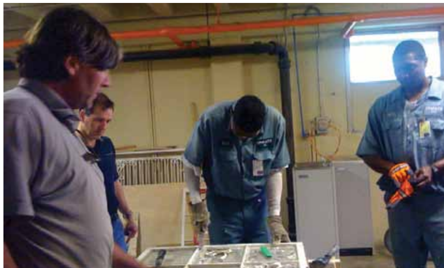
Window Restoration in Progress
