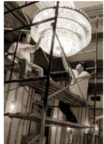
Interior Restoration in Progress
